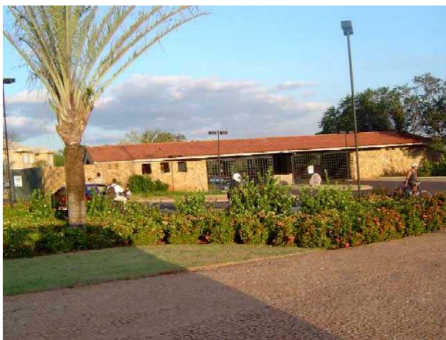
Figura 97. Muros e guarita do Condomínio Country Village
