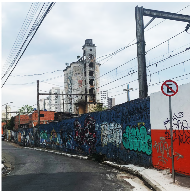
moinho central, silos
