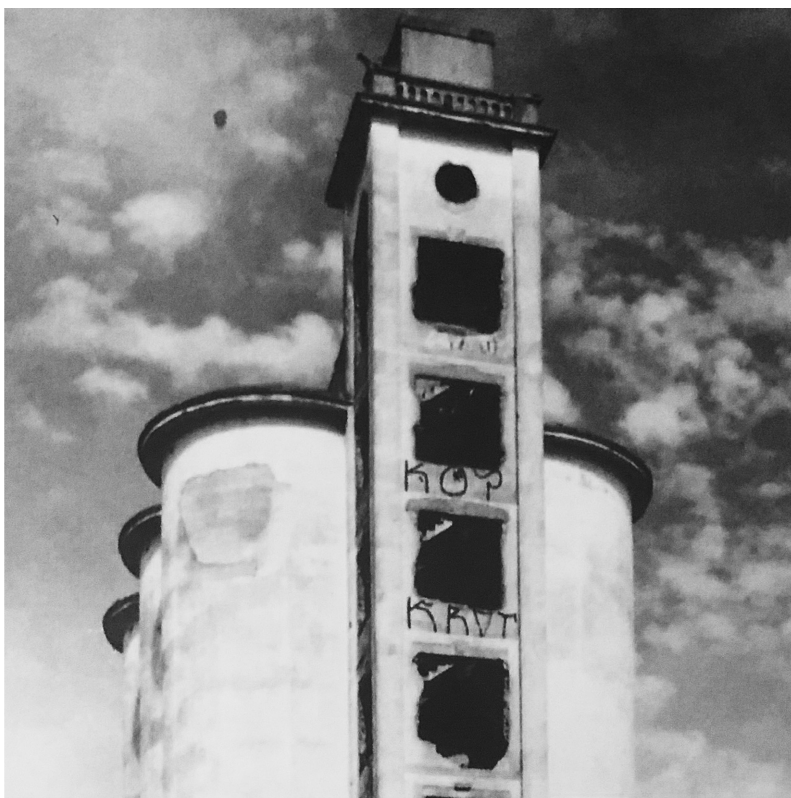
moinho central, silos
